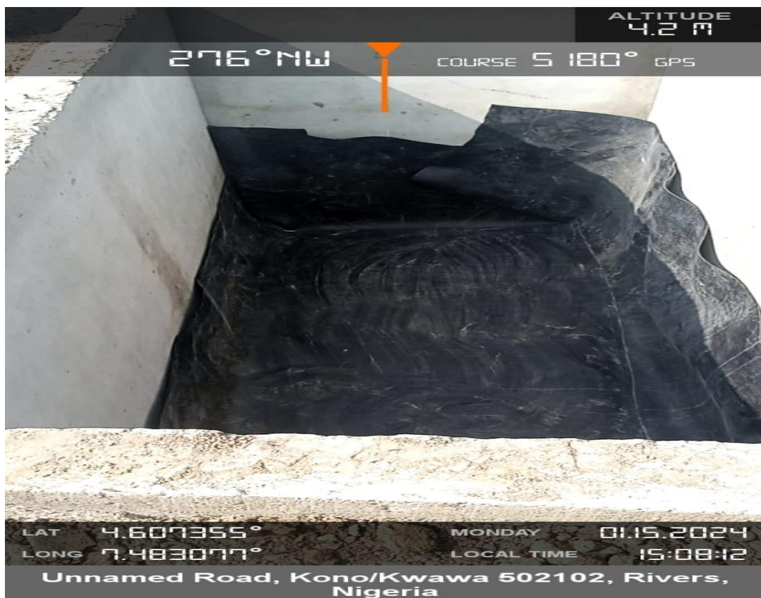
Plate 2: Placed HDPE liner in the sump
