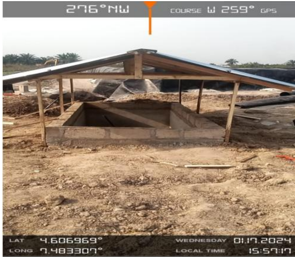
Plate 7: Completed roofing of the sump
