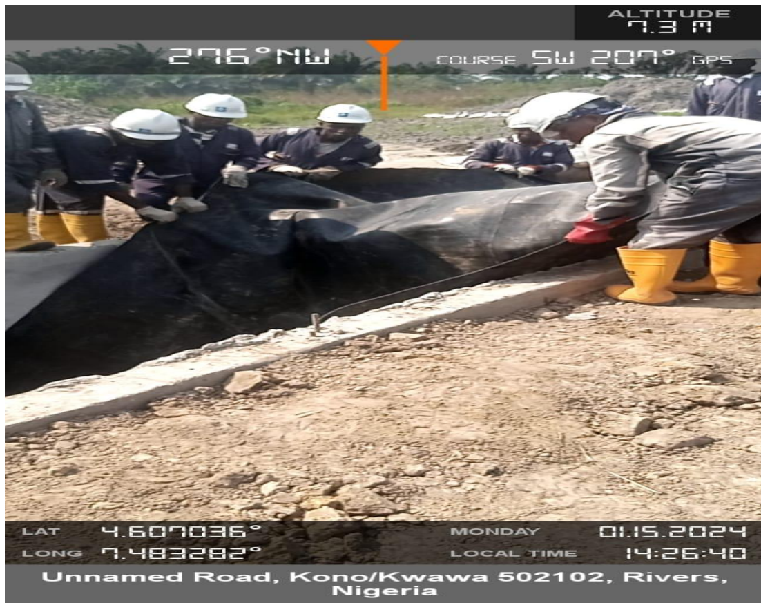
Plate 1: Placing of HDPE liner in the sump
