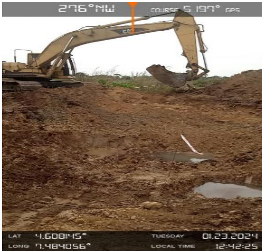
Plate 12: Removal of top soil from trenches
