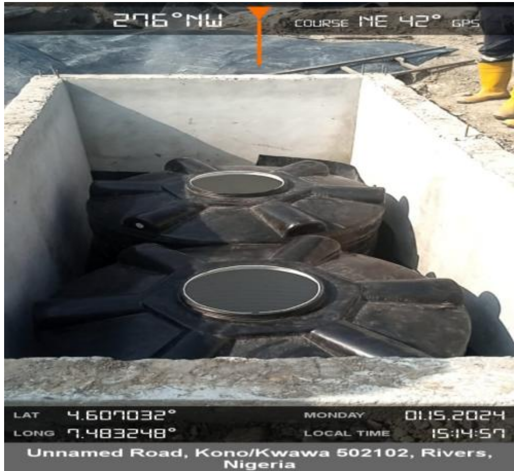
Plate 3: Gee Pee tank in the sump
